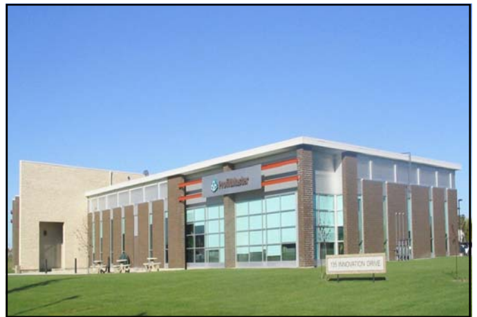
One of the Smart Park buildings at The University of Manitoba Fort Garry campus: Raymond S.C. Wan Architect Inc.; Alpha Masonry.
